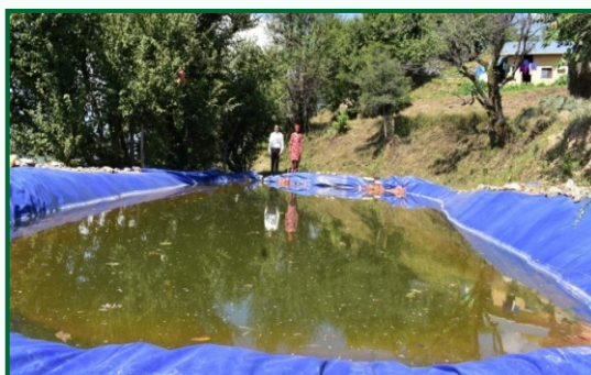
Polylined water harvesting tank, CSKHPKV, Palampur
